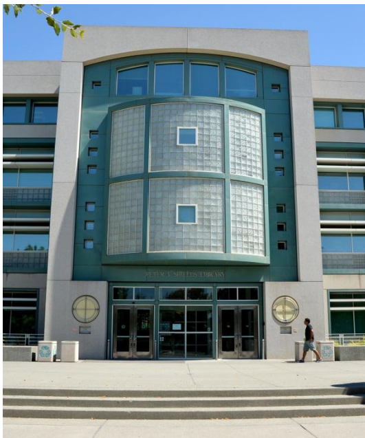
Figure 3. Simon Martin-Vegue Winkelstein Moris, Architects. Addition to Shields Library, UC Davis (1990), entrance detail.
